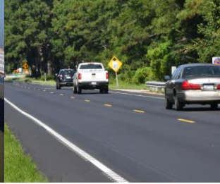
More Paving & Safety Projects
